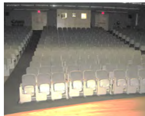
Existing steep slope of seating aisle
